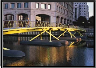
Fig. 5 West India Quay Footbridge, United Kingdom
