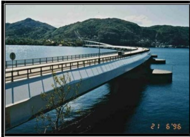
Fig. 4 Nordhordland Floating Bridge, Norway
