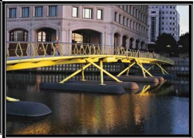
Fig. 5 West India Quay Footbridge, United Kingdom
