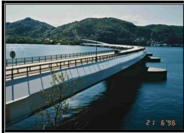
Fig. 4 Nordhordland Floating Bridge, Norway
