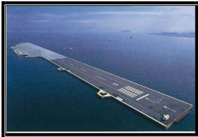
Fig. 15 Mega-Float in Tokyo Bay, Japan (Photo courtesy of SRCJ)
