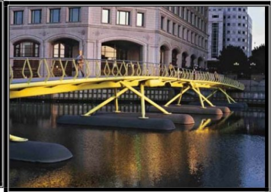
Fig. 5 West India Quay Footbridge, United Kingdom
