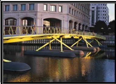
Fig. 5 West India Quay Footbridge, United Kingdom
